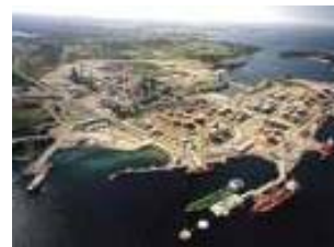
Statoil Mongstad Norway - 40 MWth Chilled Ammonia - Gas
