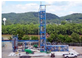
Dow Chemical Co. USA, West Virginia Advanced Amines - Coal
